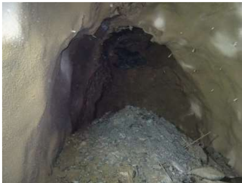
Figure 4.9 - Collapse at Ch.0+555, 11th February 2016
