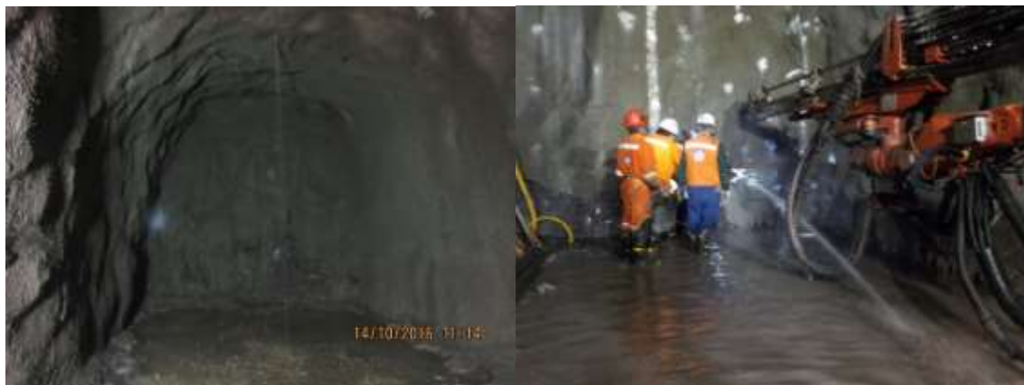
Figure 4.3 - Water inflows at chainage 1+401.8 (a) and 1+509.4 (b) in the Colimapu Formation
