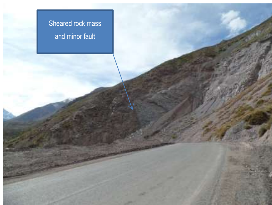
Figure 3.1 - Access road to the camp site with major disturbance of the rock mass – east side of Yeso valley south of Las Cortaderas
