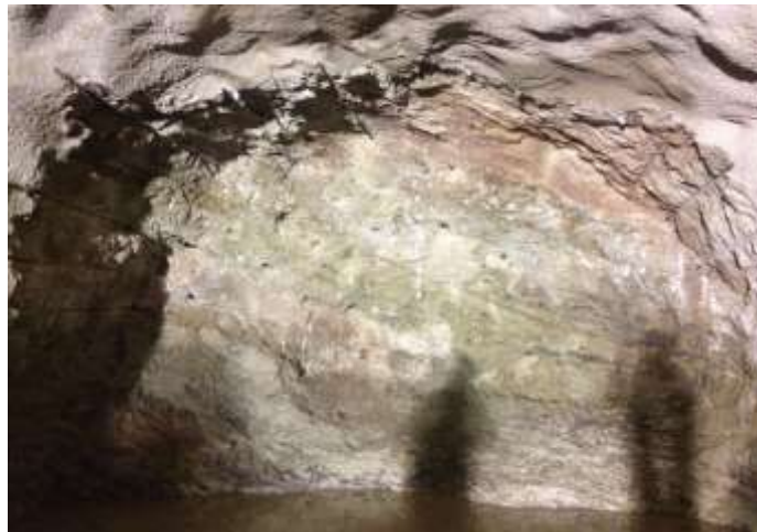
Figure 4.10 - Chainage 0+211.8 metamorphic sandstone (inflows of 130l/min experienced at the face)
