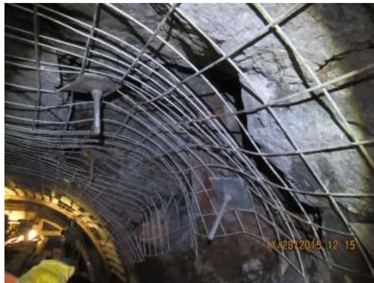
Figure 4.4 - Overbreak due to individual blocks failing at Chainage 13+438
