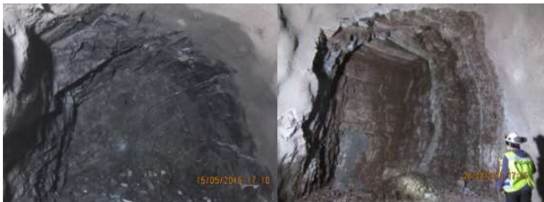
Figure 4.2 - Overbreak in andesites (a) and limestones (b) of the Lo Valdes-Colimapu Formations
