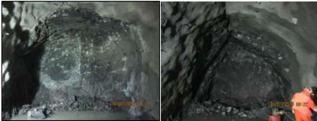
Figure 4.1 (a) and (b). - Overbreak in Rio Damas Sandstone due to joints parallel to tunnel axis (a) and in the Lo Valdes Formation in limestone (b)
