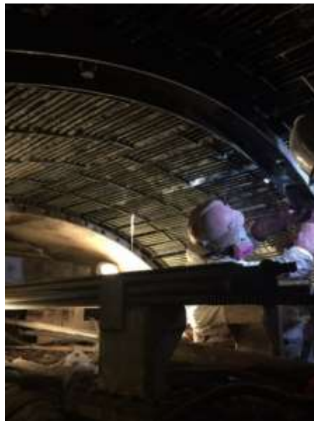
Figure 4.6 - McNally roof support system installed immediately behind the TBM cutterhead
