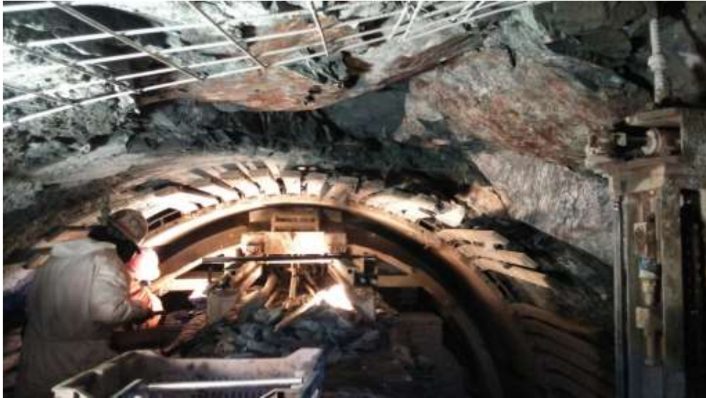
Figure 4.5 - Slabbing and block failures in the crown at Chainage 13+293
