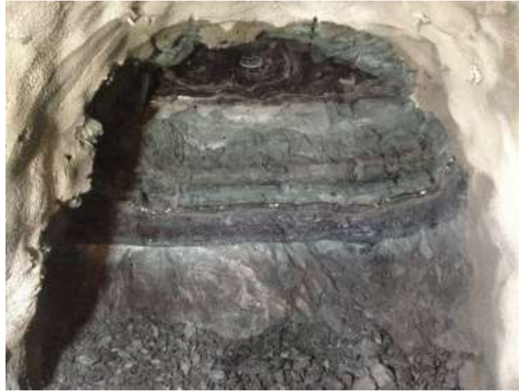
Figure 4.8 - Chainage 0+542.9 Sub-horizontal contact between the andesite and volcanic tuff
